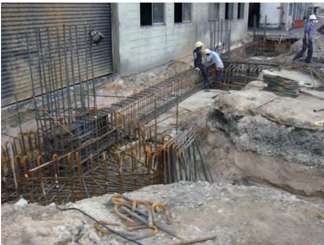
Foundation of Product Storage Tank – Thai Tokai Carbon Product
