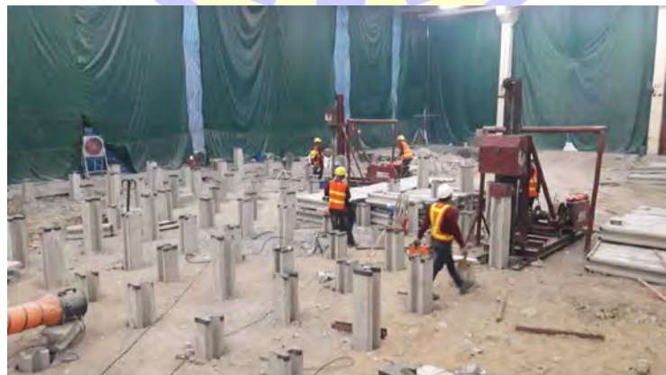
Bridgestone /Constuction of Mold stock and Chemical Room
